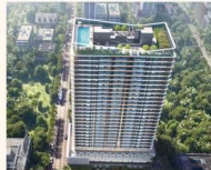
Oak West Residency 1&2&3 Bedroom Westlands (under construction)
