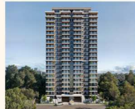
Venus Oak Residency 4 Bedroom Lavington (under construction)
